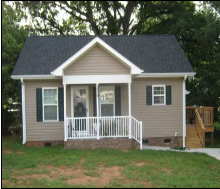
279 Moore Street, Mills Mill
