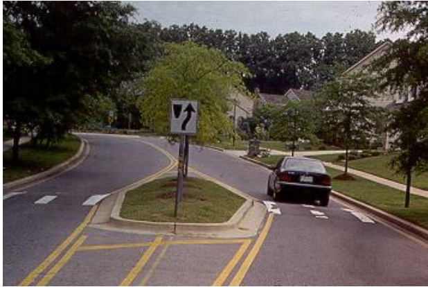
Raised Crosswalk with Center Island
