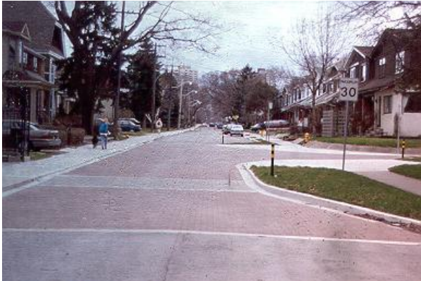
Raised Intersection with Neckdown
