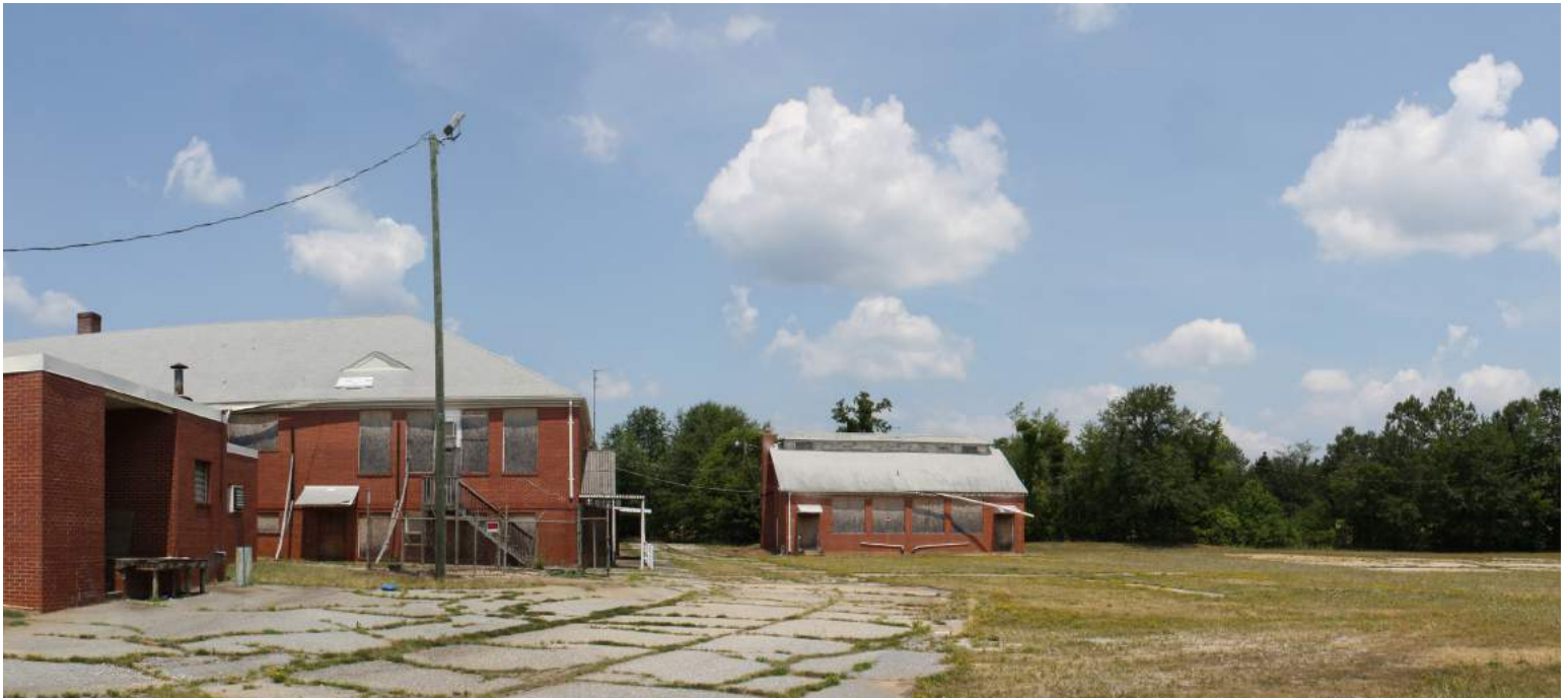
Historic Berea School Property.
