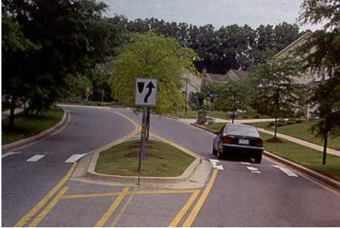
Raised Crosswalk with Center Island
