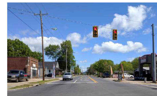
Woodside Avenue is a nearby example of an effective lane reduction project that improves both pedestrian and vehicular safety.
