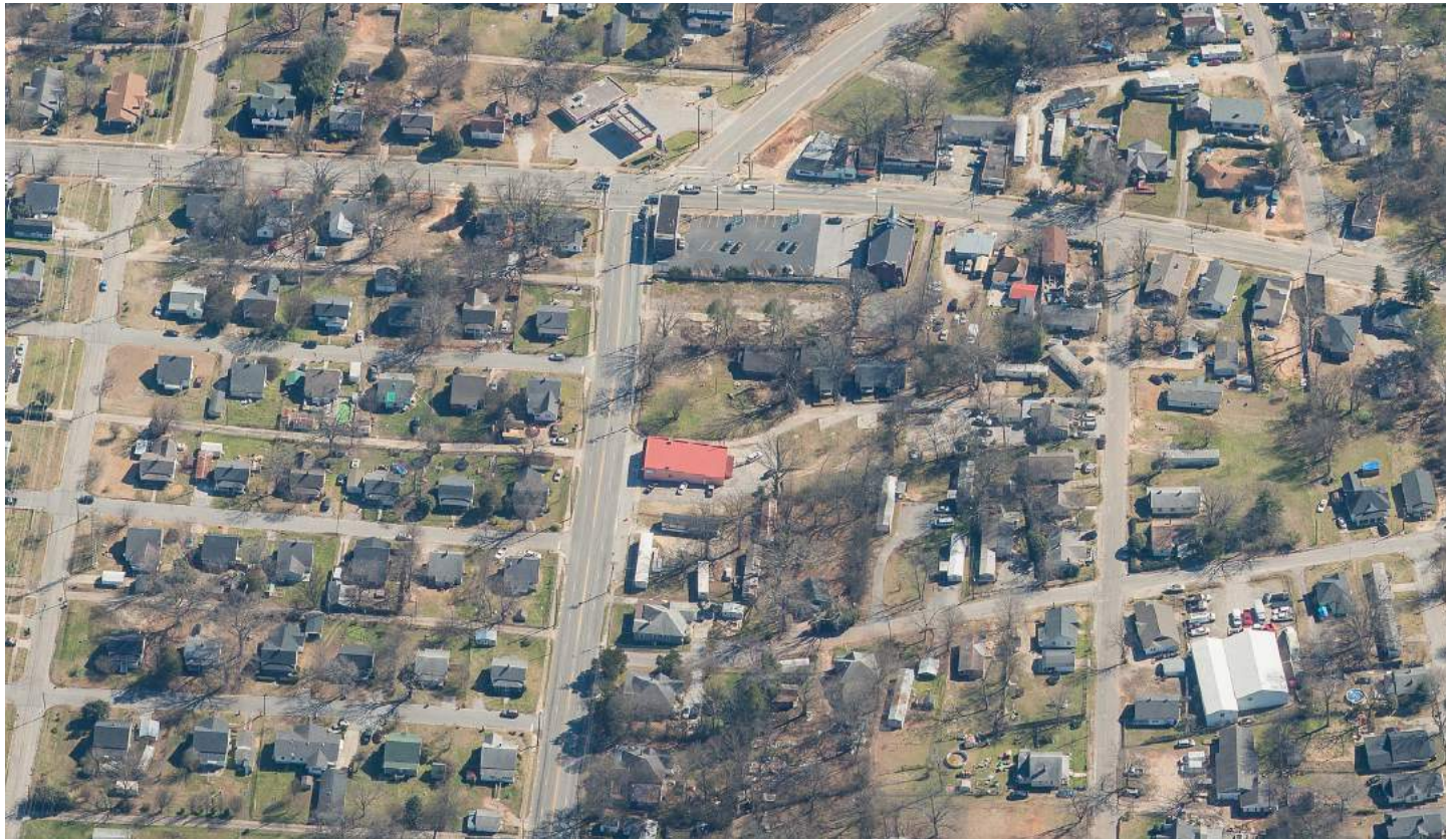
Oblique photo of Woodside Avenue
