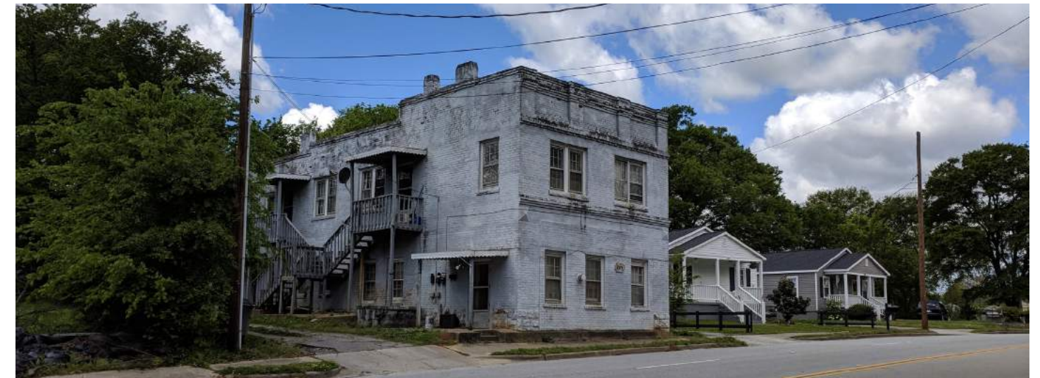
A dilapidated multi-family housing complex in City View
