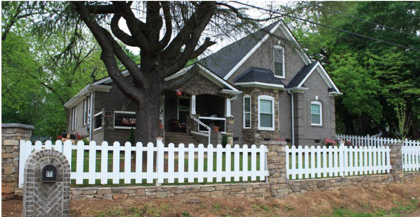
New construction in City View
