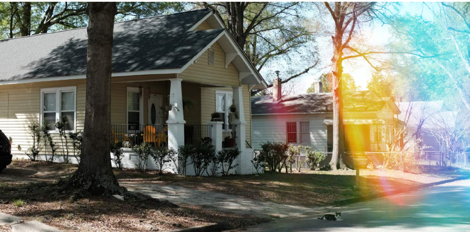
Mill homes on Beattie Street
