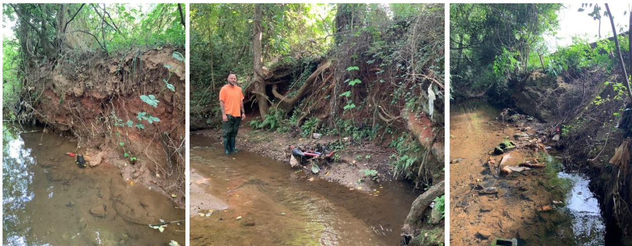
Figure 2.1 - Existing conditions along the unnamed tributary.
