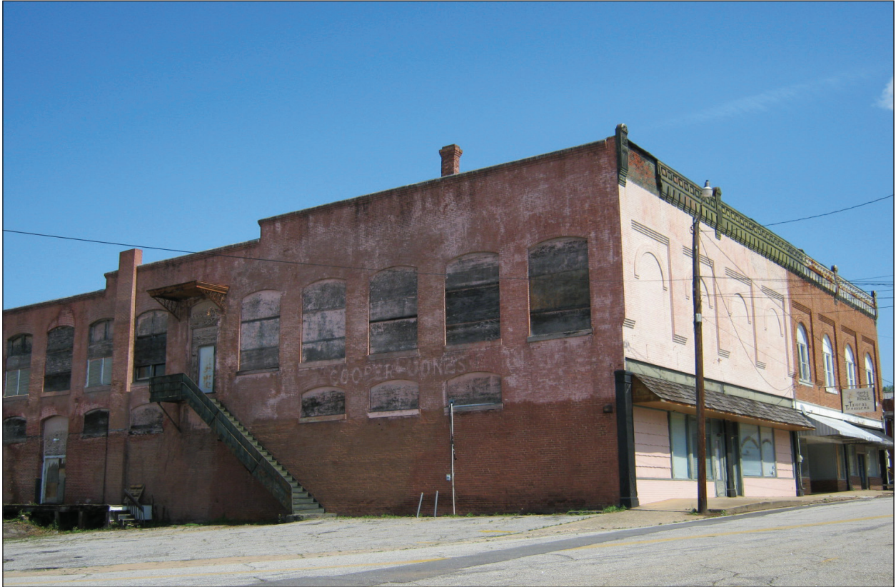
Figure 5.41 Resource 3269, a commercial building in the Piedmont Mill Village, south oblique.
