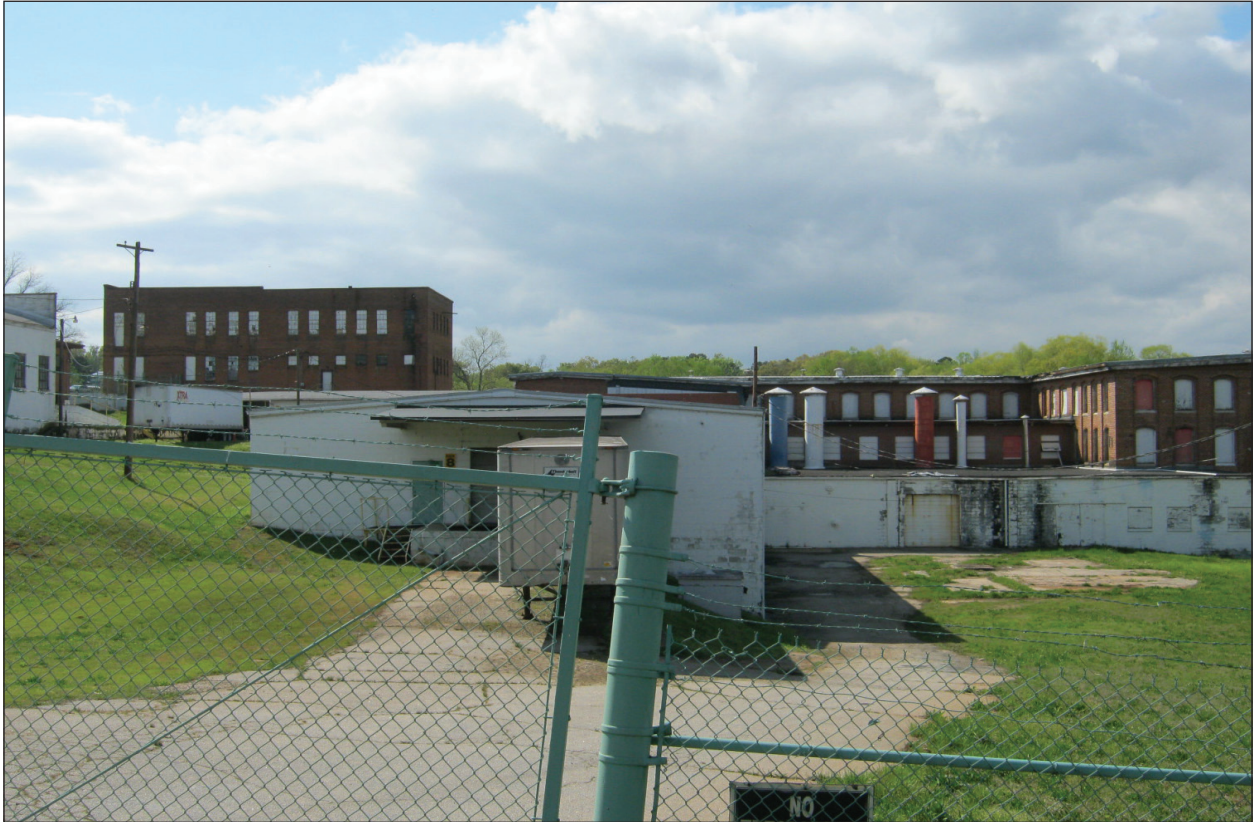
Figure 5.33 Resource 3207, Overview of Conestee Mill, facing northwest.
