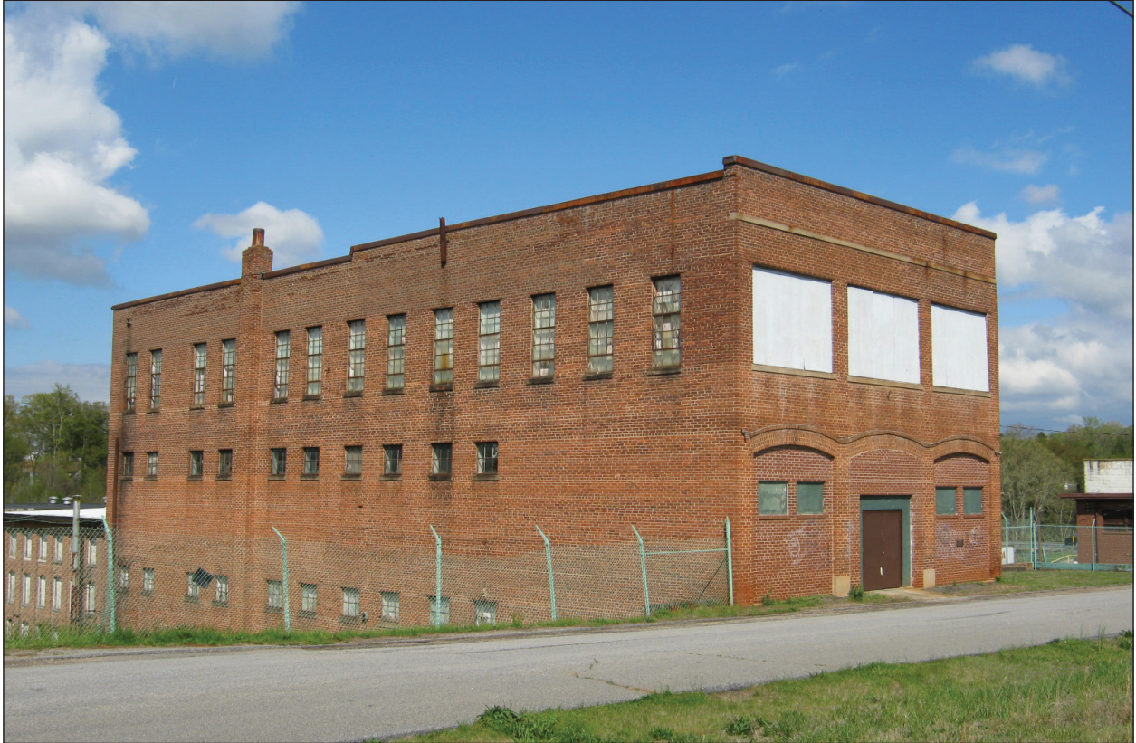
Figure 5.34 Resource 3893, Conestee Mill community store and post office, west oblique.
