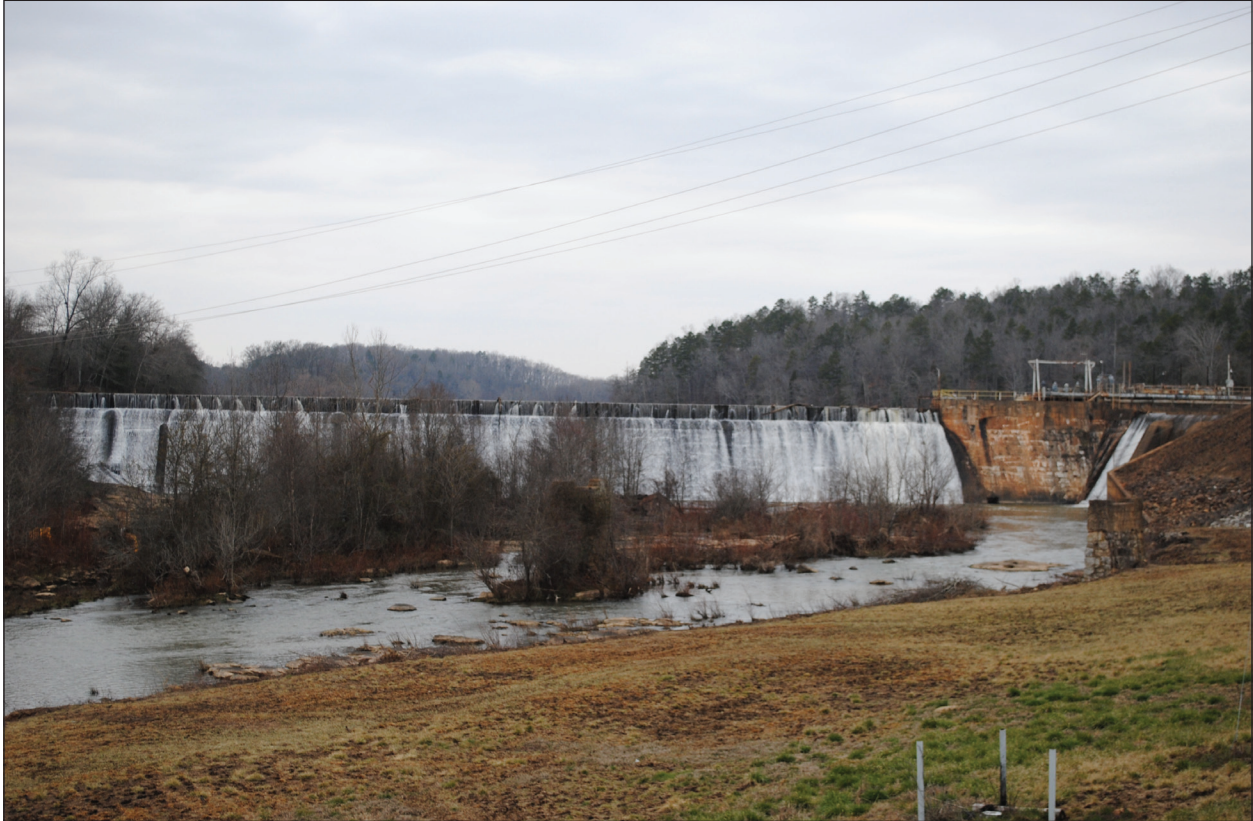
Figure 5.2 Resource 2836, Holiday Bridge dam, facing northwest.
