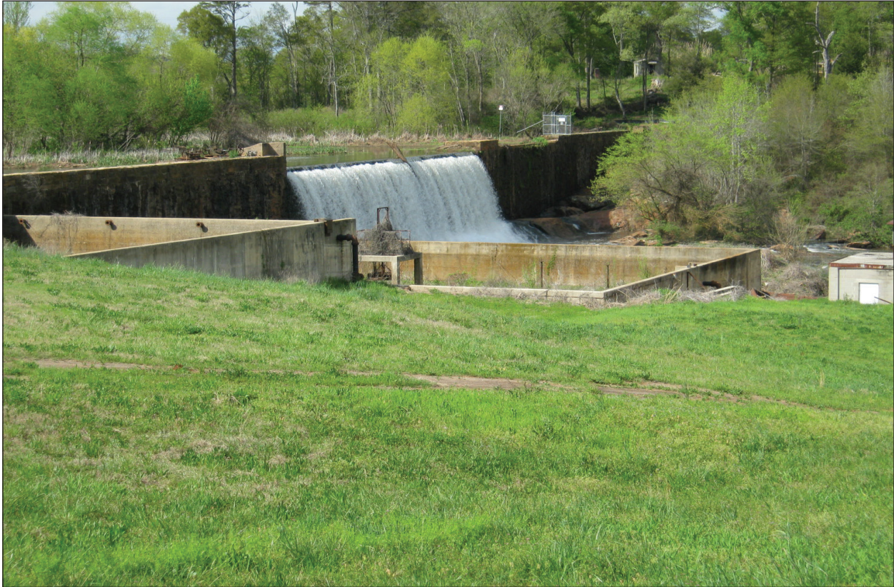
Figure 5.35 Resource 3899, Conestee dam, facing north.
