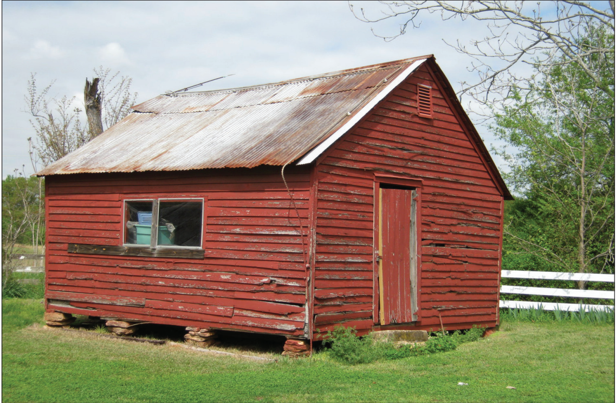
Figure 5.17 Resource 3885, shed, southwest oblique.
