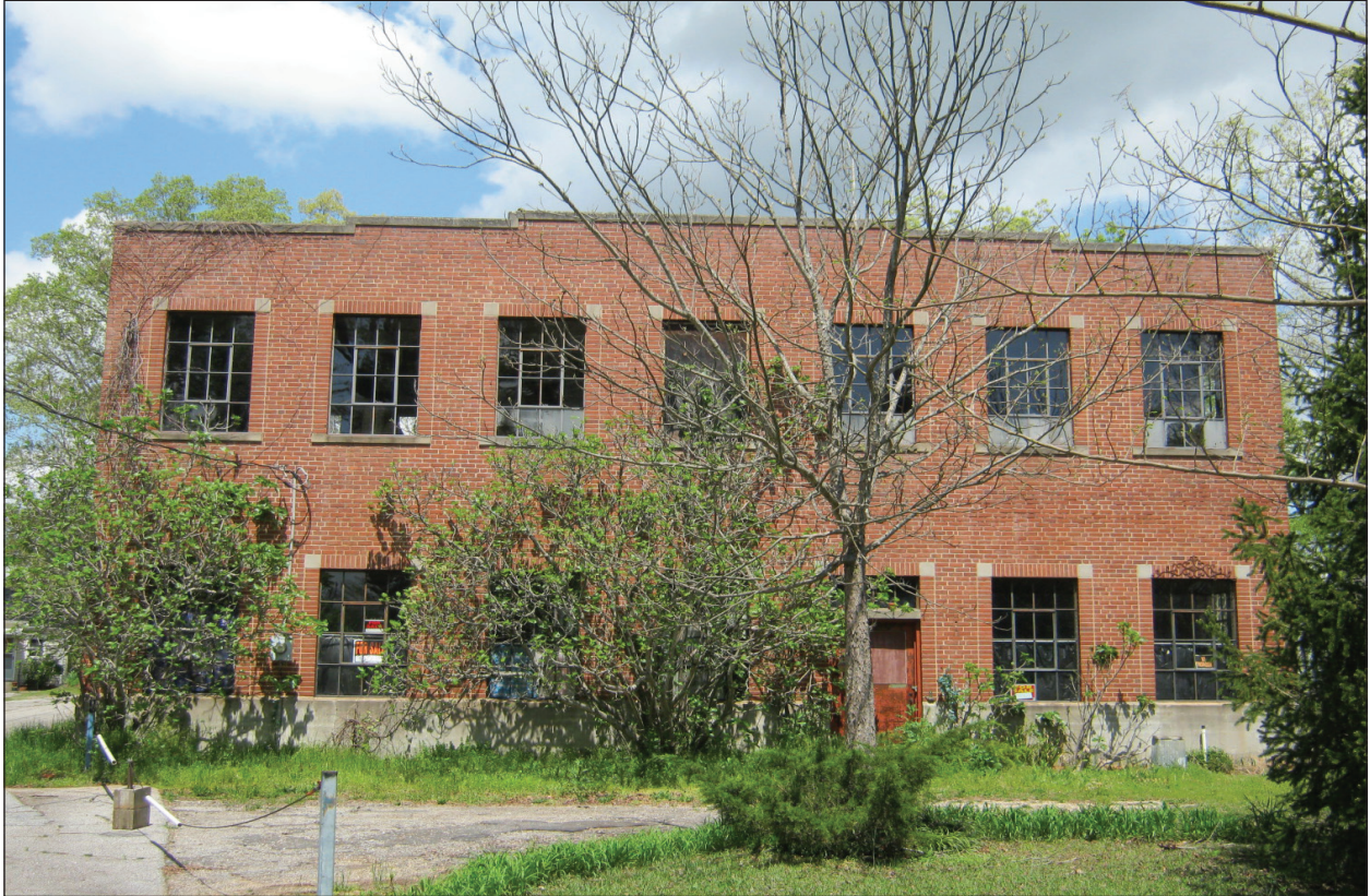
Figure 5.42 Resource 3279, an institutional building in the Piedmont Mill Village, south elevation.
