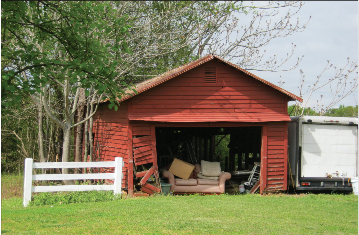
Figure 5.16 Resource 3883, shed, south elevation.
