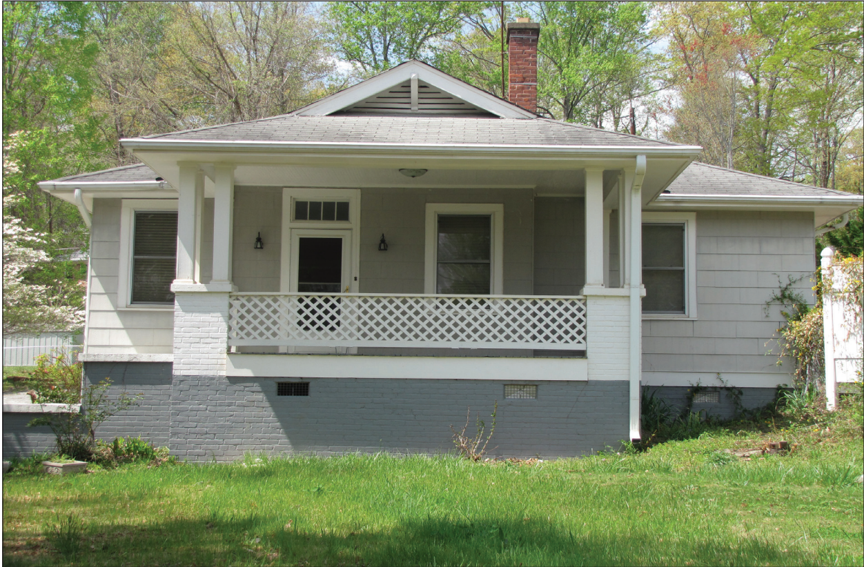
Figure 5.51 Resource 3492, a typical house in the Slater Mill Village, southeast elevation.
