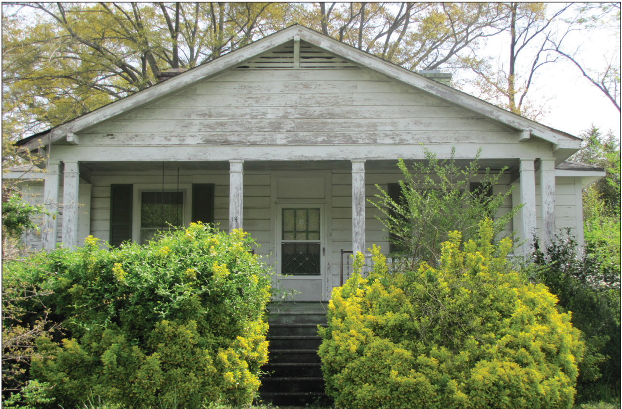
Figure 5.50 Resource 3476, a typical house in the Slater Mill Village, southwest elevation.
