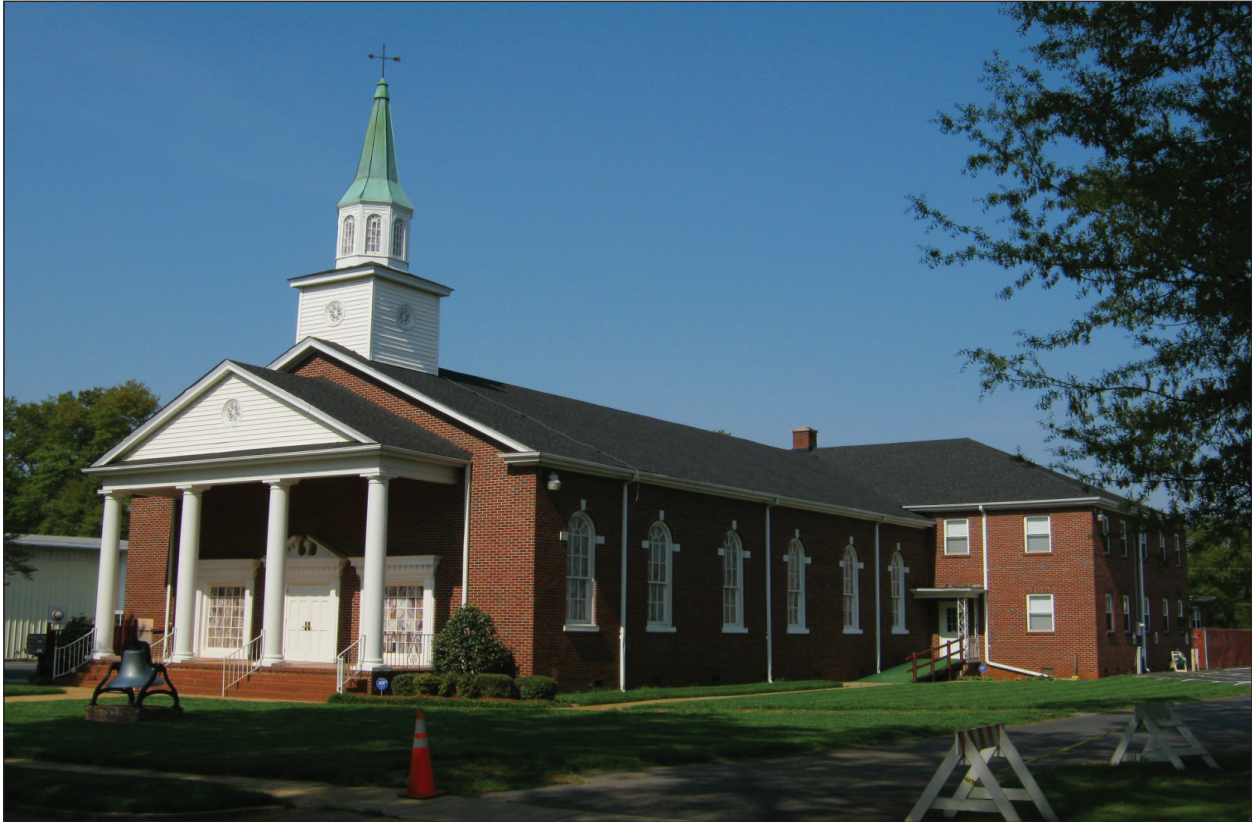
Figure 5.55 Resource 3253, Union Bleachery Baptist Church, southeast elevation.
