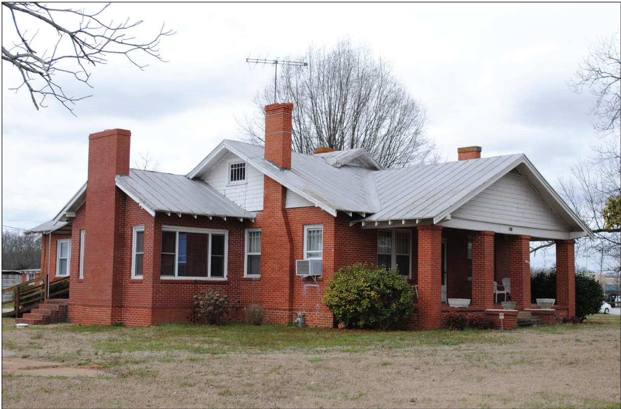
Figure 4.10 View of Resource 2907, example of a Craftsman-style house.
