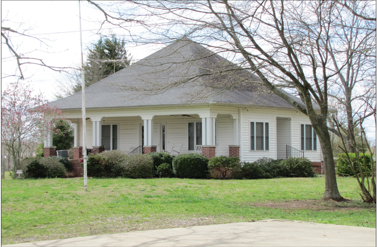
Figure 4.19 Resource 3052, an example of the pyramidal house type in Greenville County.
