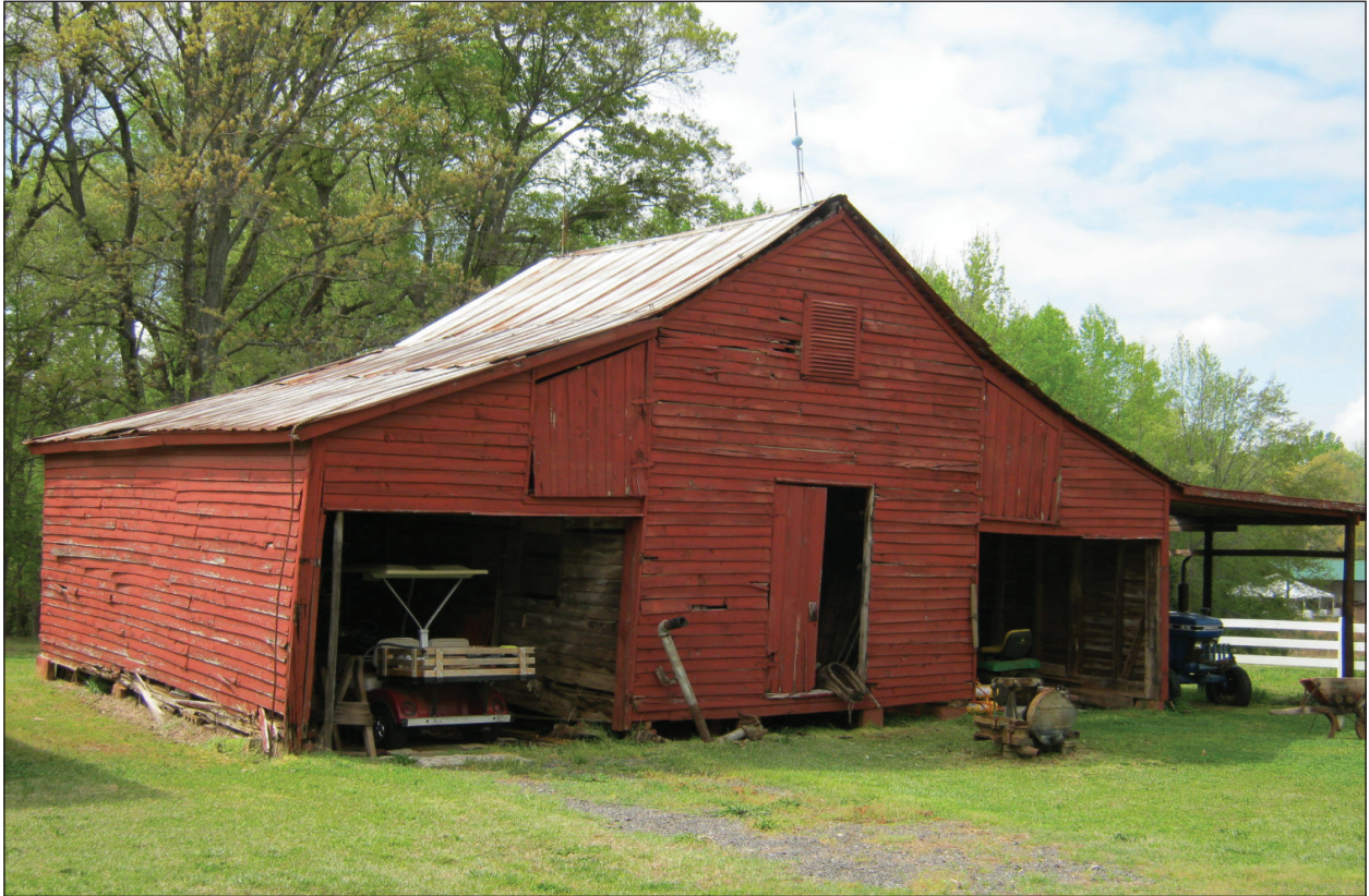
Figure 5.14 Resource 3879, barn, southeast elevation.
