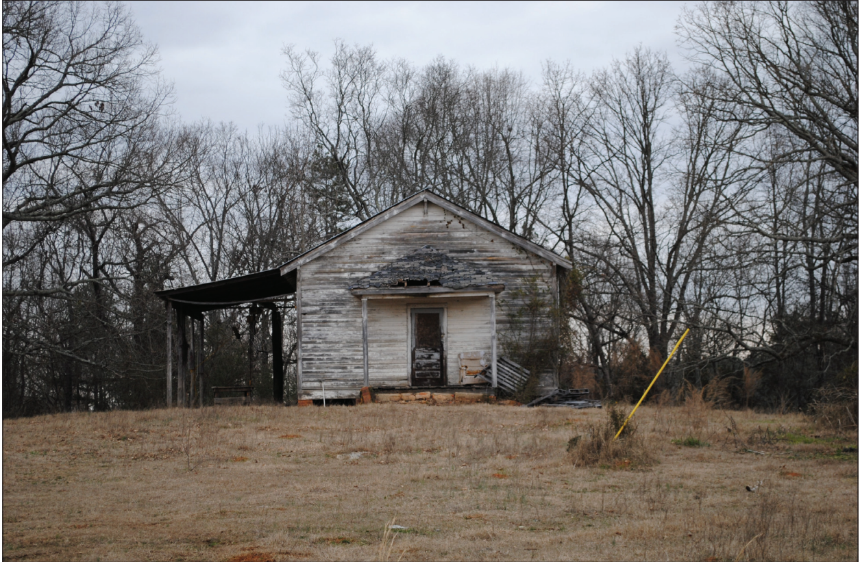
Figure 4.25 View of Resource 2837, a rural one-room schoolhouse.
