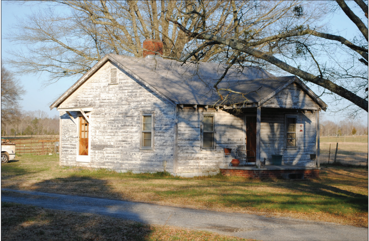
Figure 4.15 Resource 2875, an example of a massed-plan side-gable house type in Greenville County.
