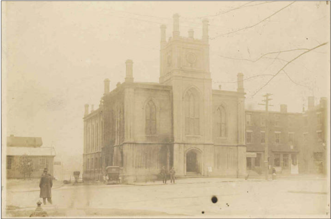
Figure 2.10 Photograph of the Gothic-styled 1855 courthouse prior to demolition in 1915 (Clemson University Libraries, http://contentdm.clemson.edu/u/?spg,56 ).
