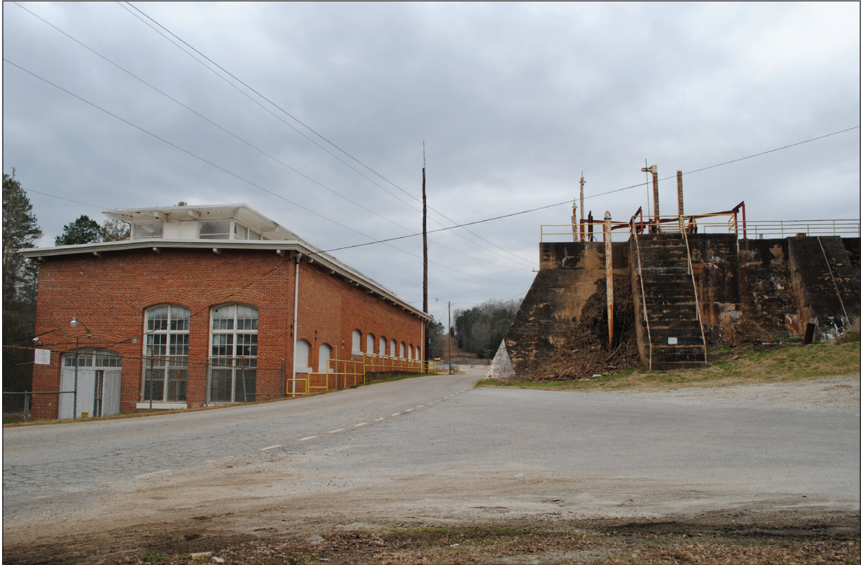
Figure 5.1 Resource 2835, Holiday Bridge hydro station.
