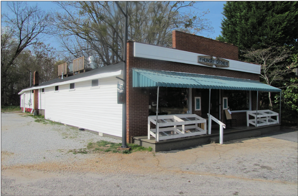
Figure 4.21 View of Resource 3296, typical freestanding commercial structure.
