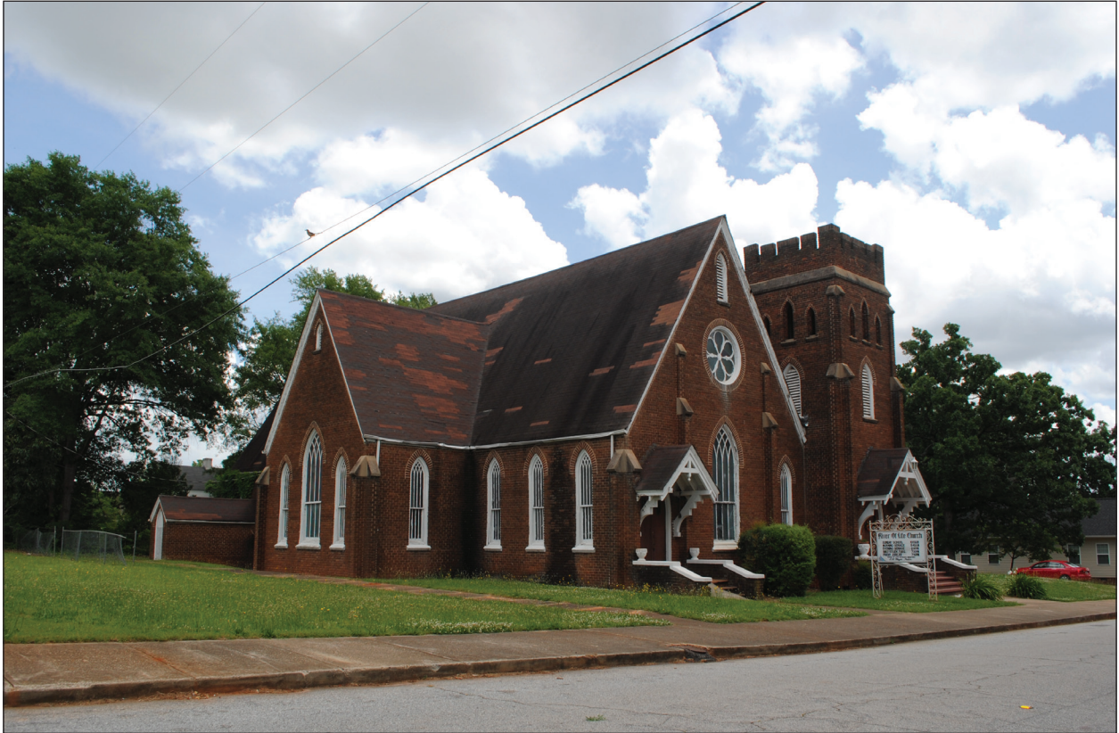
Figure 4.22 View of Resource 3799, the River of Life Church, a typical example of the Gothic Revival style.
