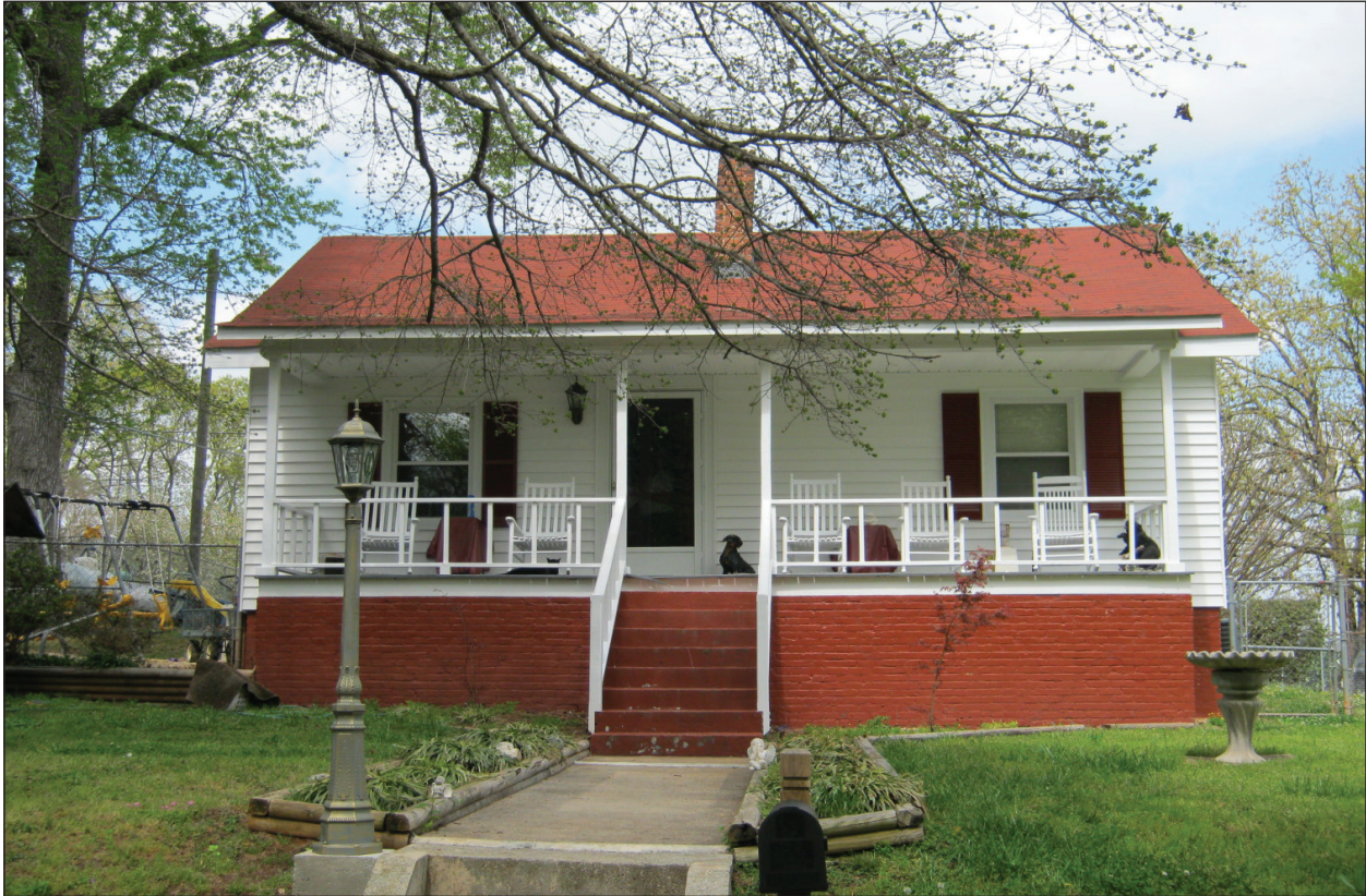
Figure 5.47 Resource 3235, a typical house in the Renfrew Bleachery Community, southwest elevation.
