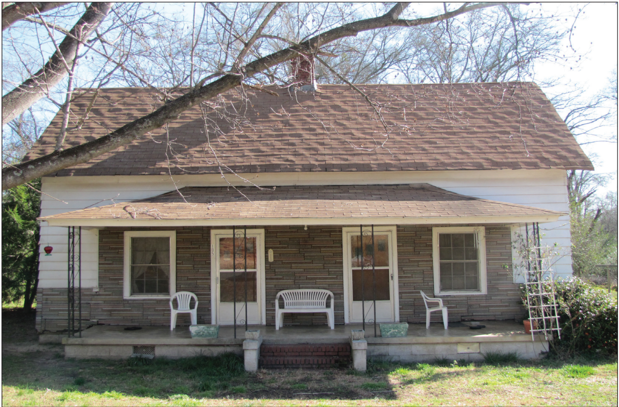
Figure 5.37 Resource 2962, a typical Fork Shoals mill house, southwest elevation.
