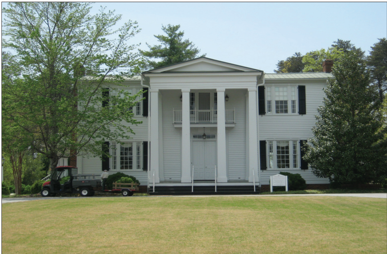
Figure 5.22 Resource 3261, northeast elevation.
