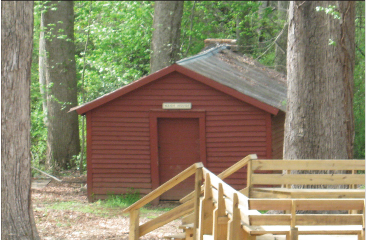
Figure 5.18 Resource 3887, wash house, southeast elevation.
