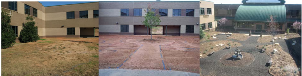
Figure 3. Before, During and After Courtyard Project Implementation.
