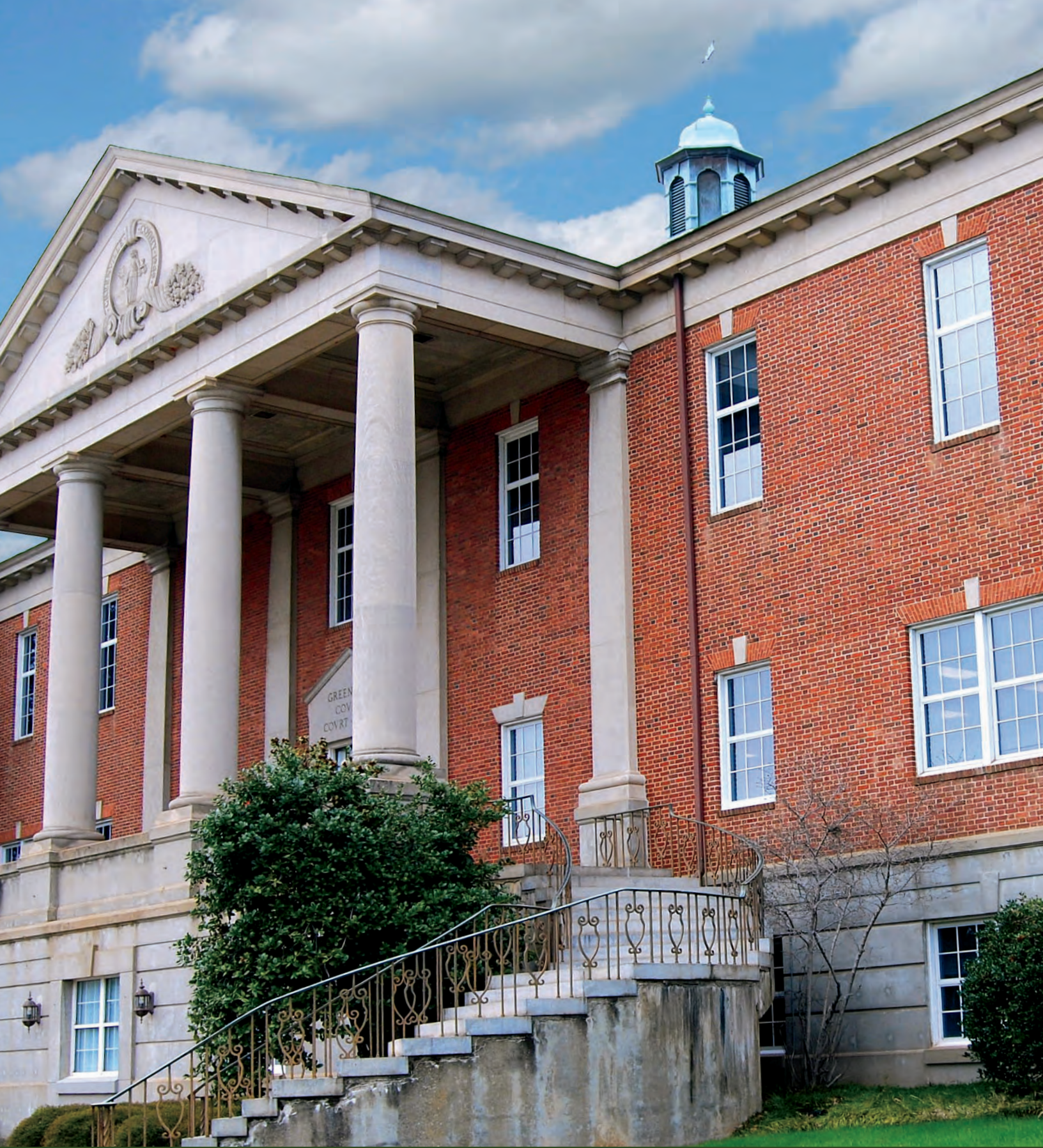
County Courthouse located at corner of Church and East North Street
