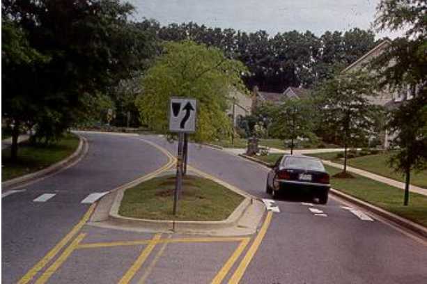
Raised Crosswalk with Center Island
